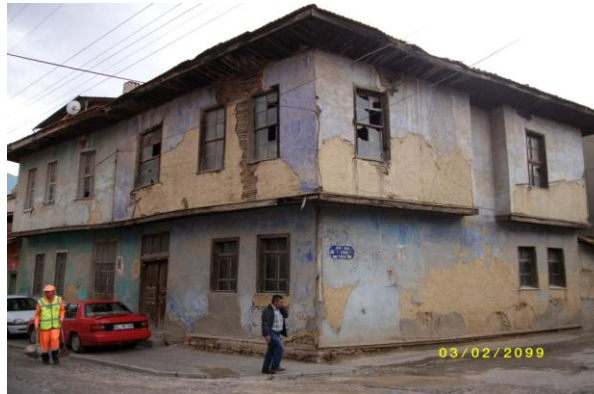
Picture 9. Işık Neighborhood, Timber Frame Construction
