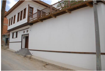
Picture 1: Dokur House, Aybey Neighborhood, Wood Frame Construction
