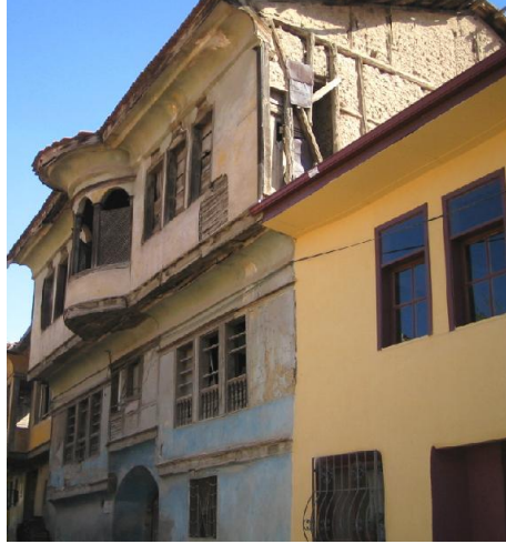
Picture 10. Ali Osman Tosun Timber Frame Construction.
