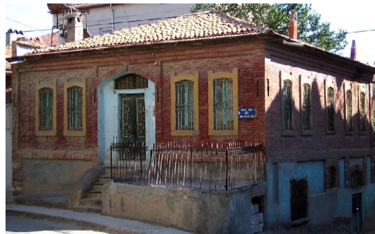
Picture 6. Masonry House in Ünalán Neighborhood.
