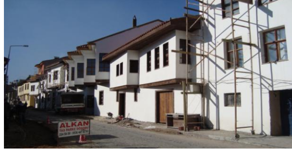
Picture 4. Timber Frame Houses
