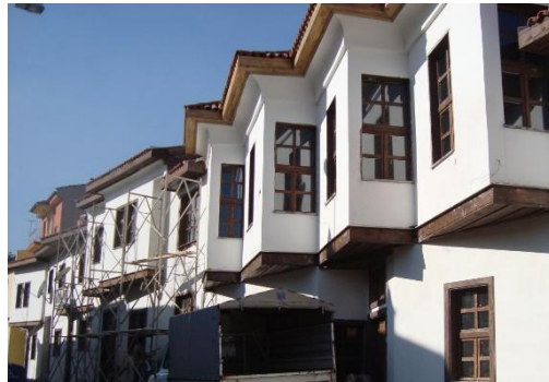
Picture 3. Timber Frame House after restoration.
