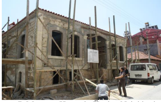
Picture 7. Masonry House in Ünalán Neighborhood.
