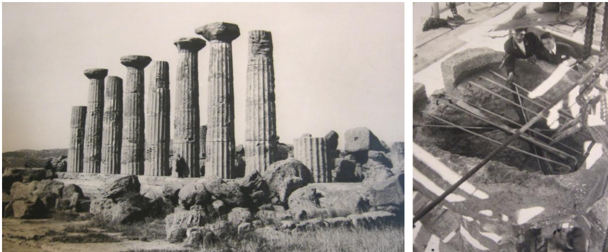
Figures 2, 3: The Heracles temple in Akragas after the eng. F. Valenti restorations (1922-1924); The capital with iron and mortar cement (in Ferrara 2010, p. 185).
