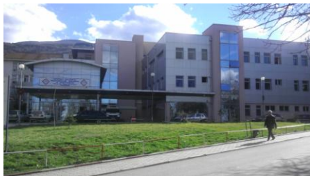
Figure 12: Regional hospital in Prizren, 2014
