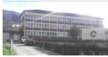
Figure 18: Regional hospital in Prizren
