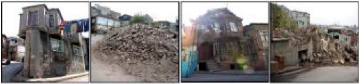
Figure 6: Demolished buildings in the Süleymaniye Region, 2009
