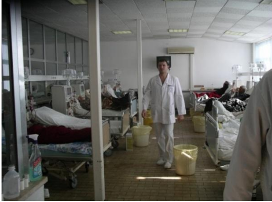
Figure 2: Executing works in spaces with patients and medical personnel
