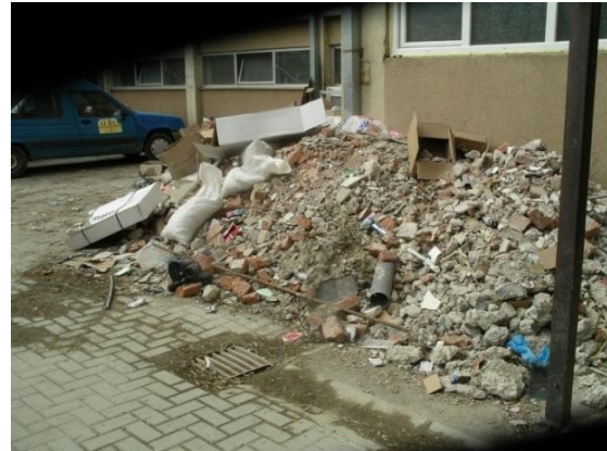
Figure 2: Construction waste put on the hospital yard
