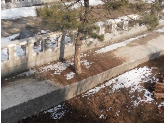
Figure 1: Not professional utilization of materials illustrated by putting concrete around trees
