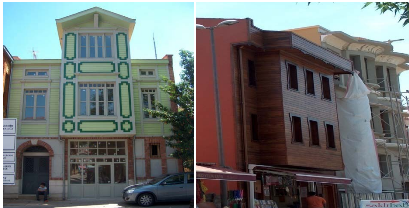
Figure 11 Insides concrete, exteriors seem traditional timber frame buildings, Eyüp (Istanbul)
