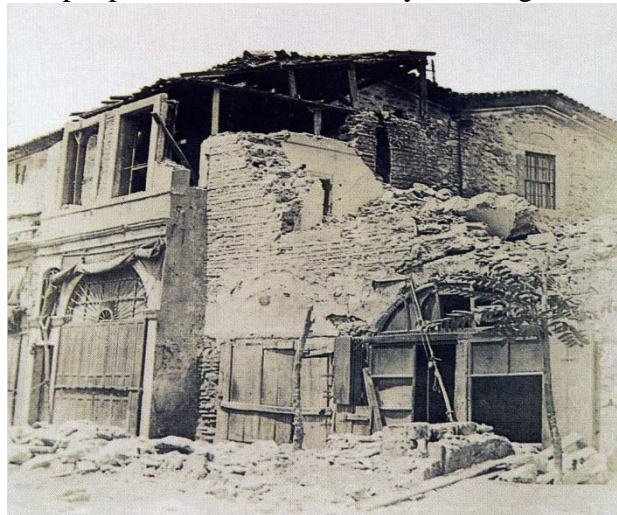
Figure 3 After 1794 Big Earthquake, ruins of stones [8]
