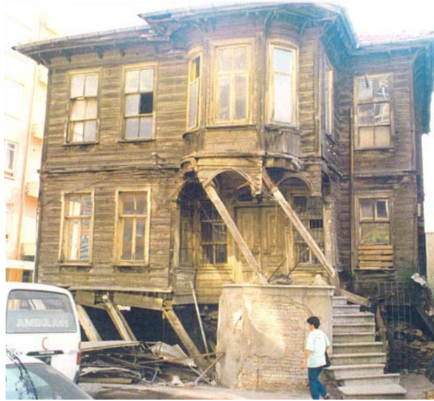
Figure 4 Half demolished timber buildings after Düzce Earthquake [3]
