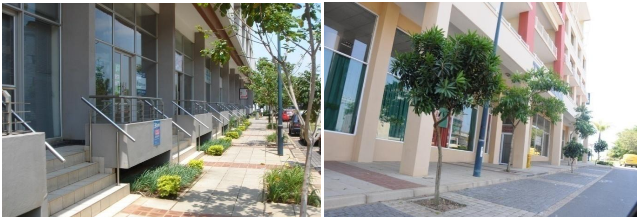
Fig. 13: Retail units on the main boulevard, empty and screened with blinds. The levels were raised to allow natural ventilation of the parking basements underneath. The raised levels give a sense of privacy towards the ground floor units, not necessarily desired in a retail context (28 October 2011).
