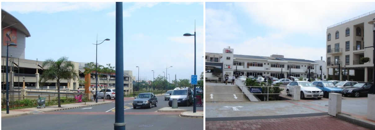
Fig. 17: The Gateway Shopping Centre's relationship to Twilight Street. The parking structure is located on this edge and in turn affects the interface with the street edge. The traffic is predominantly vehicle oriented.
