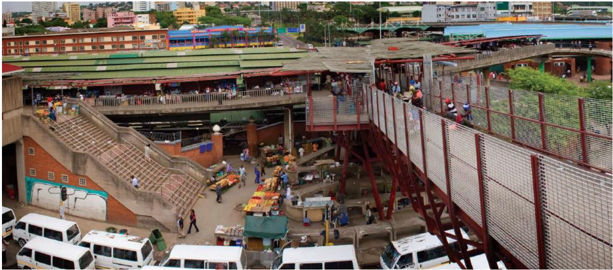
Fig. 12: The pedestrian bridge with a robust permeable balustrade to enhance passive surveillance and increase security. (Dobson et al, 2009:41)
