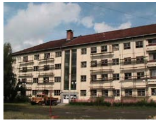
Figure 14. Beginning of retrofit
