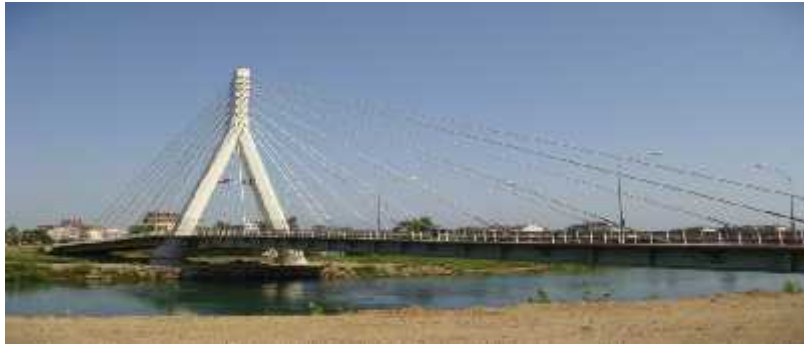
Figure 1 Manavgat Cable-Stayed Bridge
