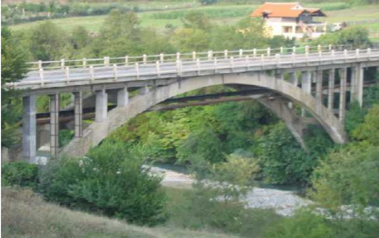
Fig.6 - Bridge in Burrel-Albania, reinforcement of vertical column
