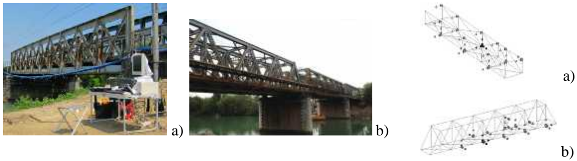
Figure 10 Instrumentation installation and setup configurations on reticular bridges.
