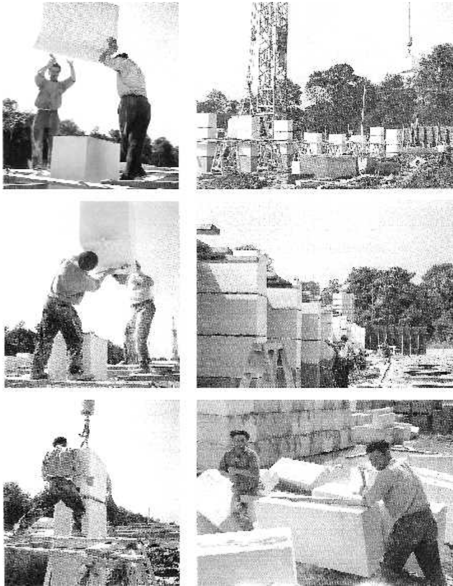
Figure 5: Assembly techniques of stone blocks on Pouillon's construction sites
