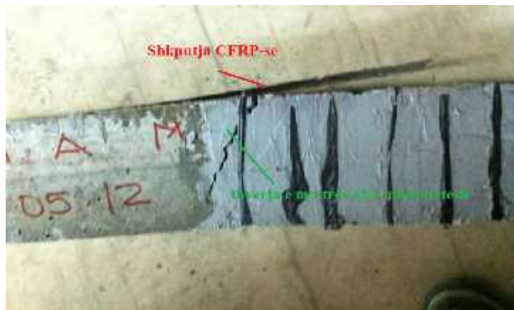
Fig.5.2-delaminate of the CFRP in Set A/beam 3
