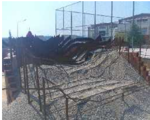
Figure 4 Formation of the concrete surfaces
