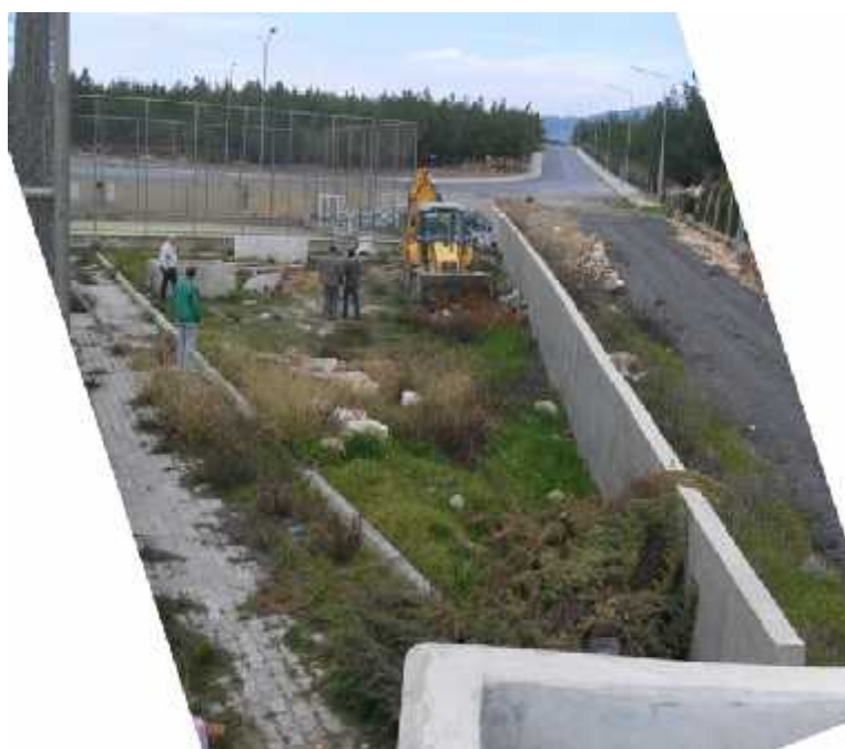
Figure 2 The initial sight of the construction sight.
