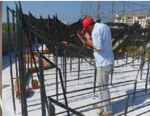
Figure 3b Placing of the sections
