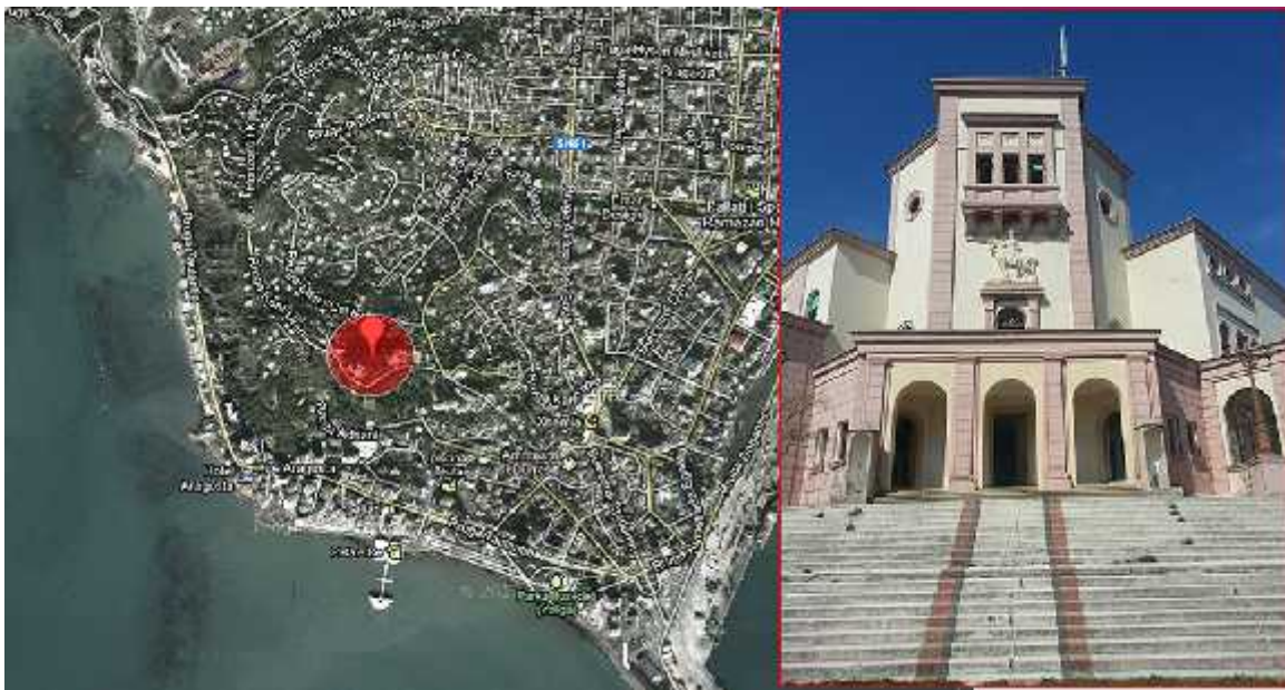
Figure 3. Aerial view of the villa (left), main façade (south) of the villa (right)
