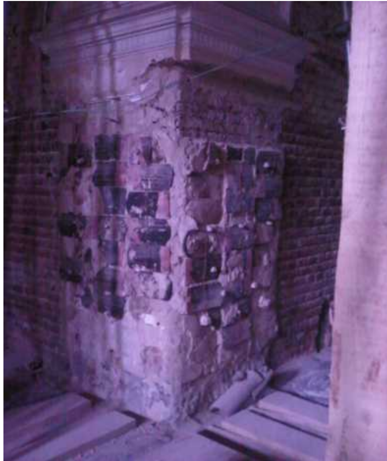
4. Historical waterproofing – with roof tiles –Károlyi Castle, Carei, Romania. (Foto Ligia Andreica)
