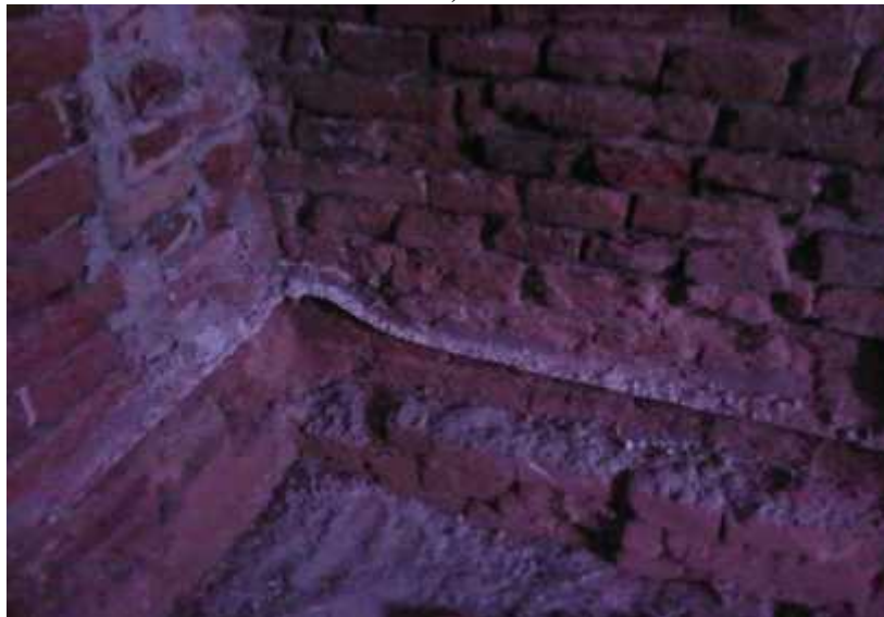
5. Contemporary waterproofing –Károlyi Castle, Carei, Romania. (Foto Ligia Andreica)
