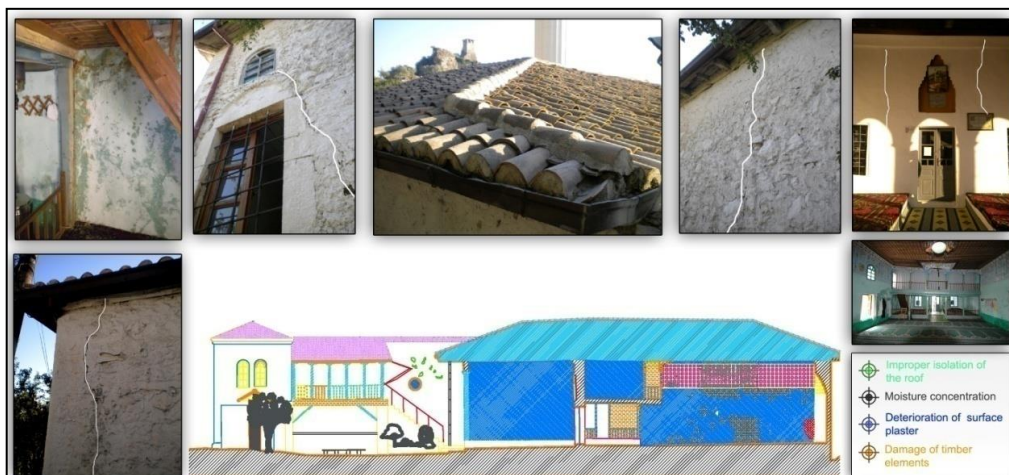
Figure 4. Inspection of structural problems of Naziresha's Mosque
