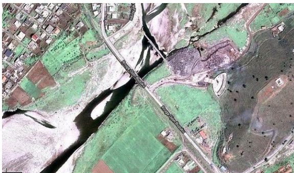
Figure 1. Aerial view of the bridge
