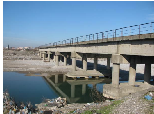
Figure 4. Piers of the bridge
