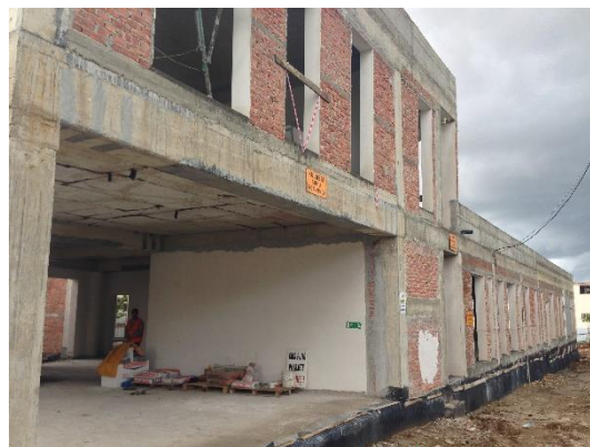
Figure 1. View of the structure
