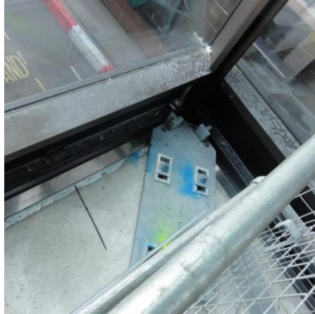
Figure 6 Unitized curtain wall corner bracket
