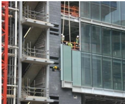
Figure 11. Unitized panel being installed by tower crane, within the edge protection [10].
