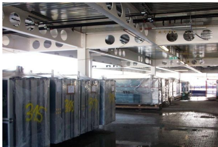
Figure 3. Element distribution and storage throughout the floors.
