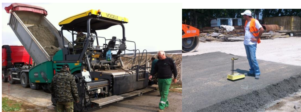
Figure 1 Left: Truck unloading onto paver and RCC laying Figure 2 Right: Fresh concrete density measured with nuclear gauge
