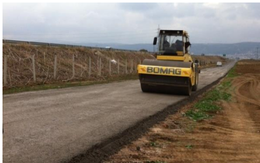
Figure 4 Roller compaction of pavement
