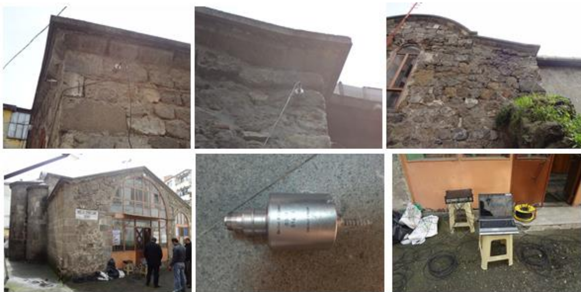
Fig. 10. The images of measurements of Molla Siyah Mosque before the restoration
