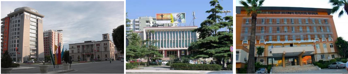
Fig 12: New building tower near the municipality. Source: Google map.
