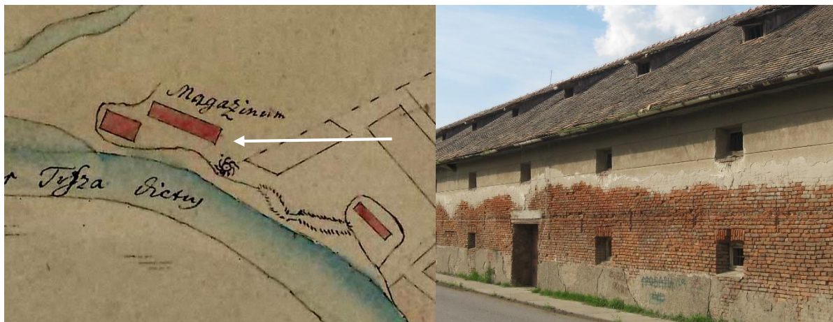
Figure 1 Grain warehouse along Tisa River, Novi Bečej
