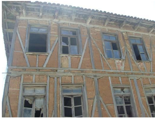
Figure 3 Wooden beams and conjunctions of earth-block structure
