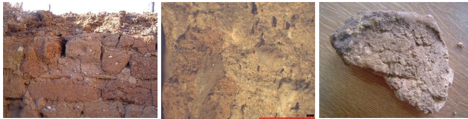
Figure 5 In situ, macroscopic and microscopic figures of structural mortars
