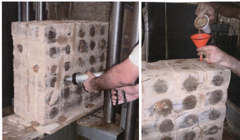
Figure 6 Grouting earth block masonry with soil based grouts
