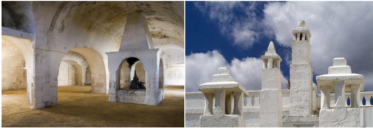
3. Detail of fireplace. 3. Detail of chimney stacks.
