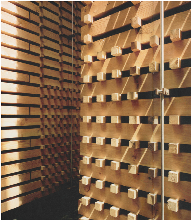
Figure 11 Peter Zumthor, Swiss Sound Box, Swiss Pavillon, Expo 2000, Hanover (1997-2000). Detail. The pavilion was constructed with 144 km of lumber with a cross-section of 20 x 10 cm, totalling 2,800 cubic metres of larch and Douglas pine from Swiss forests.
