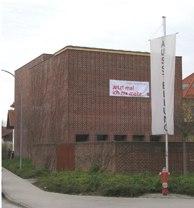
Figure 13 Valentin Bearth, Andrea Deplazes, Gallery of Contemporary Art, Marktoberdorf (1998-2000). The construction bodies of the museum are constructed of masonry in three-headed clinker exposed on both the inside and outside.
