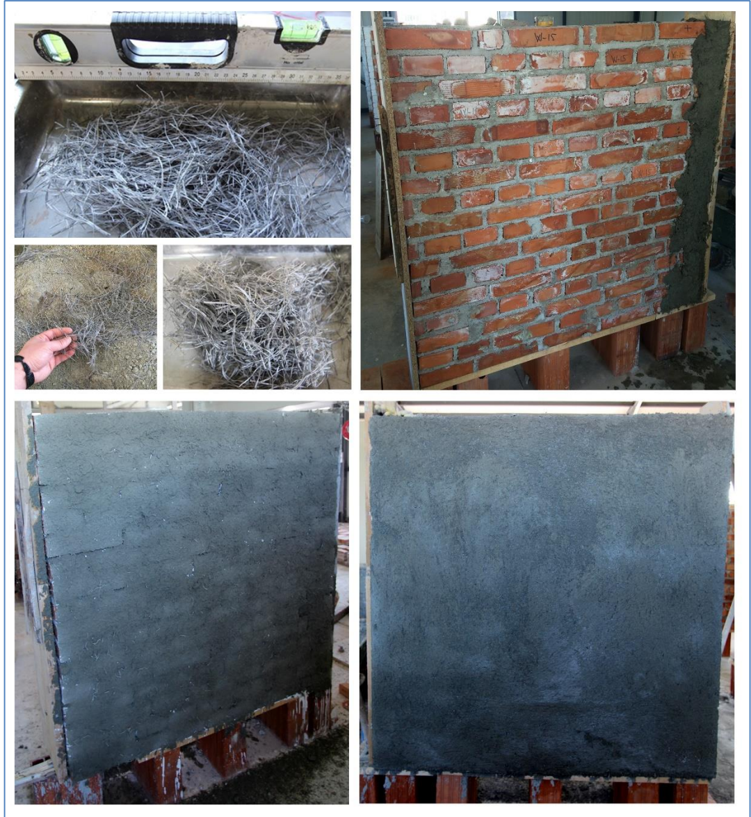
Figure 19. Plastering process with polypropylene fibres (PP).
