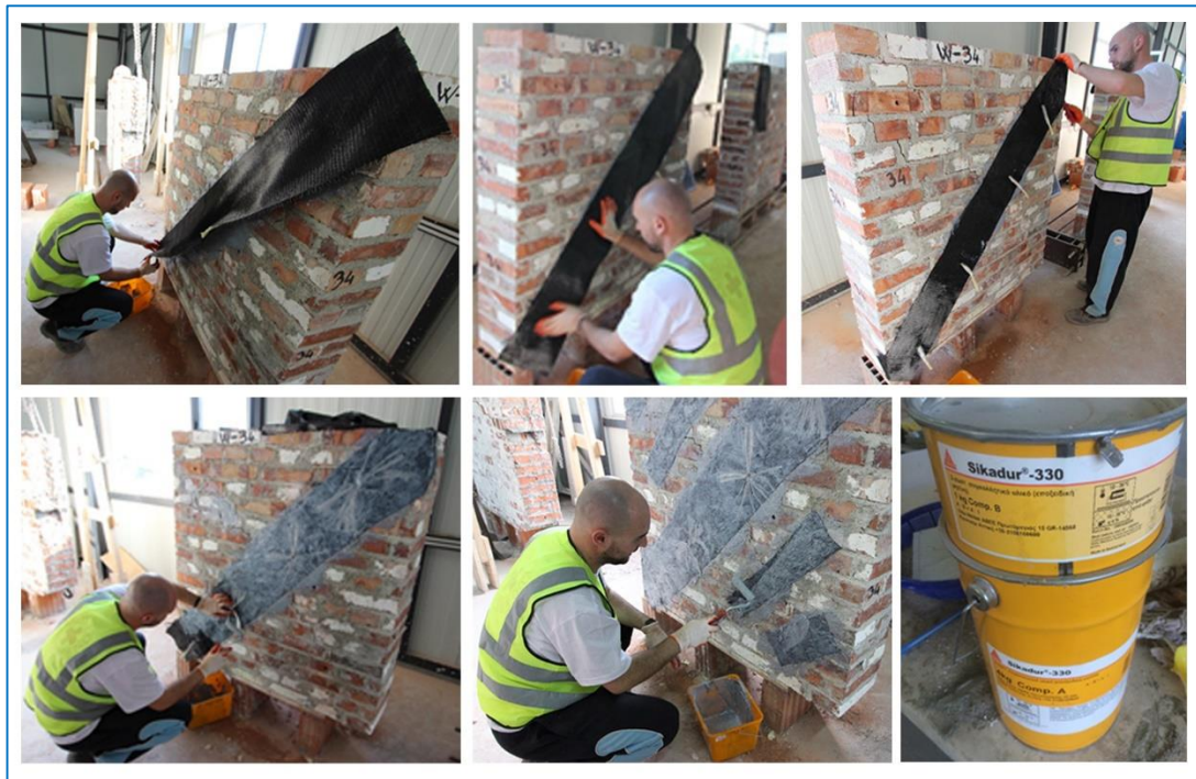
Figure 24. Repairing of the damaged walls with C-FRP (W-X-R-CFRP)
