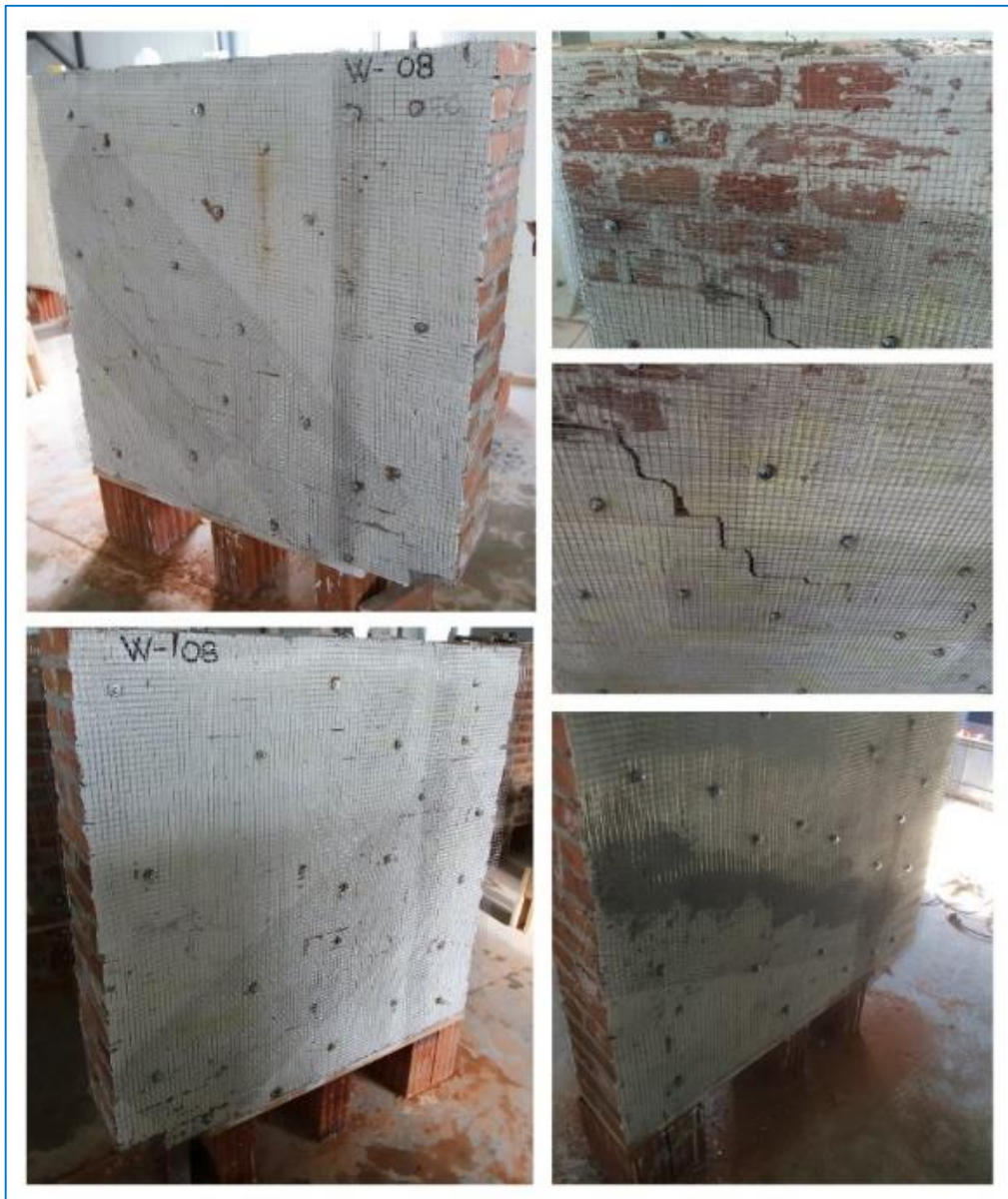
Figure 22. Repairing of the damaged walls with ferrocement jacketing (W-X-R-FC).
