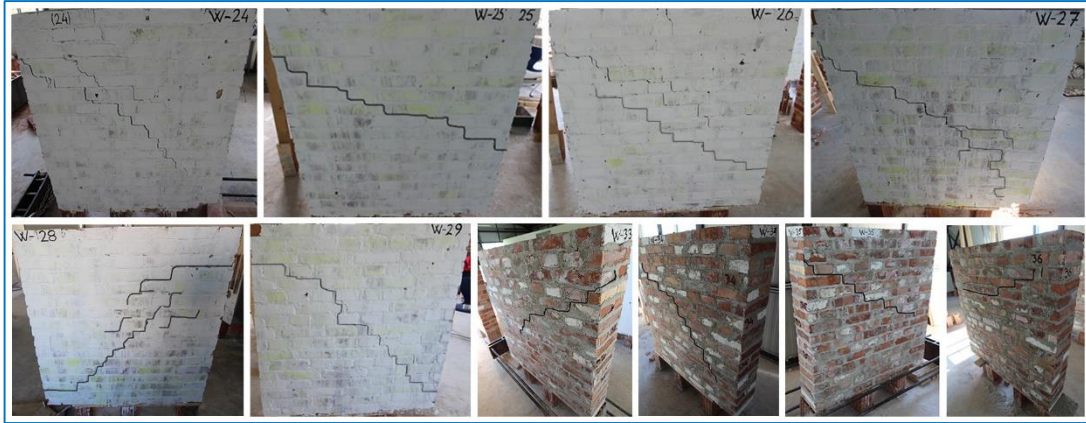
Figure 30. Failure mode of Plain walls of Series 2.
