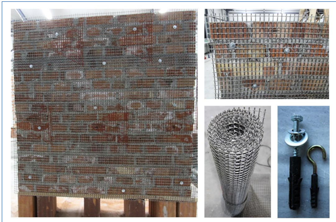
Figure 20. Plastering process with glass fibre reinforced polymer (G-FRP).
