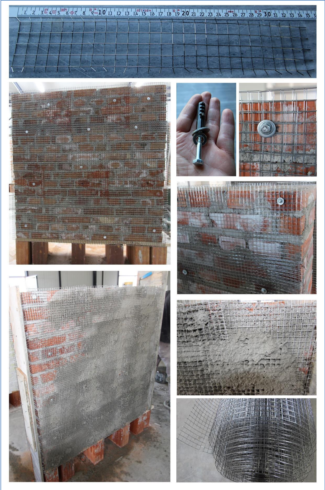
Figure 18. Plastering process with ferrocement jacketing (FC).
