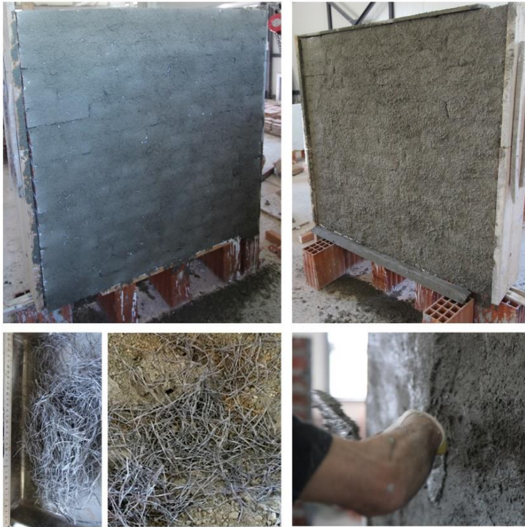
Figure 23. Repairing of the damaged walls with polypropylene fibers (W-X-R-PP).
