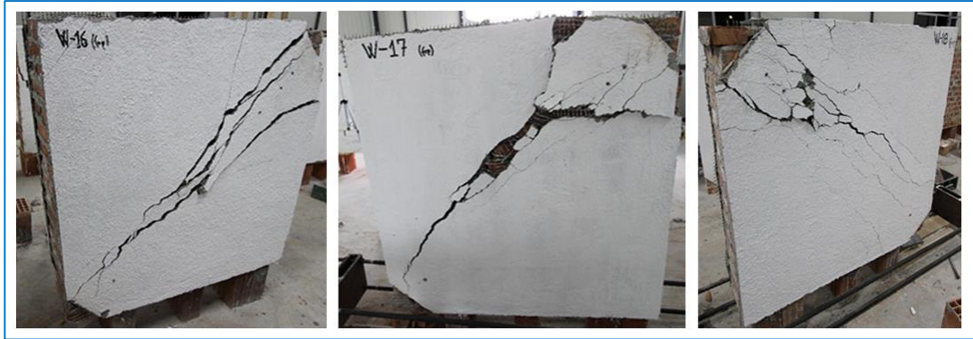
Figure 35. Failure mode of GFRP strengthened wall panels of Series 1.
