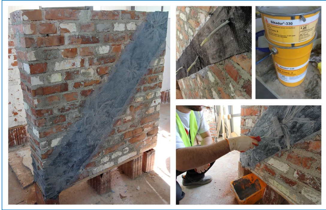
Figure 21. Application of carbon fibre reinforced polymer (G-FRP).
