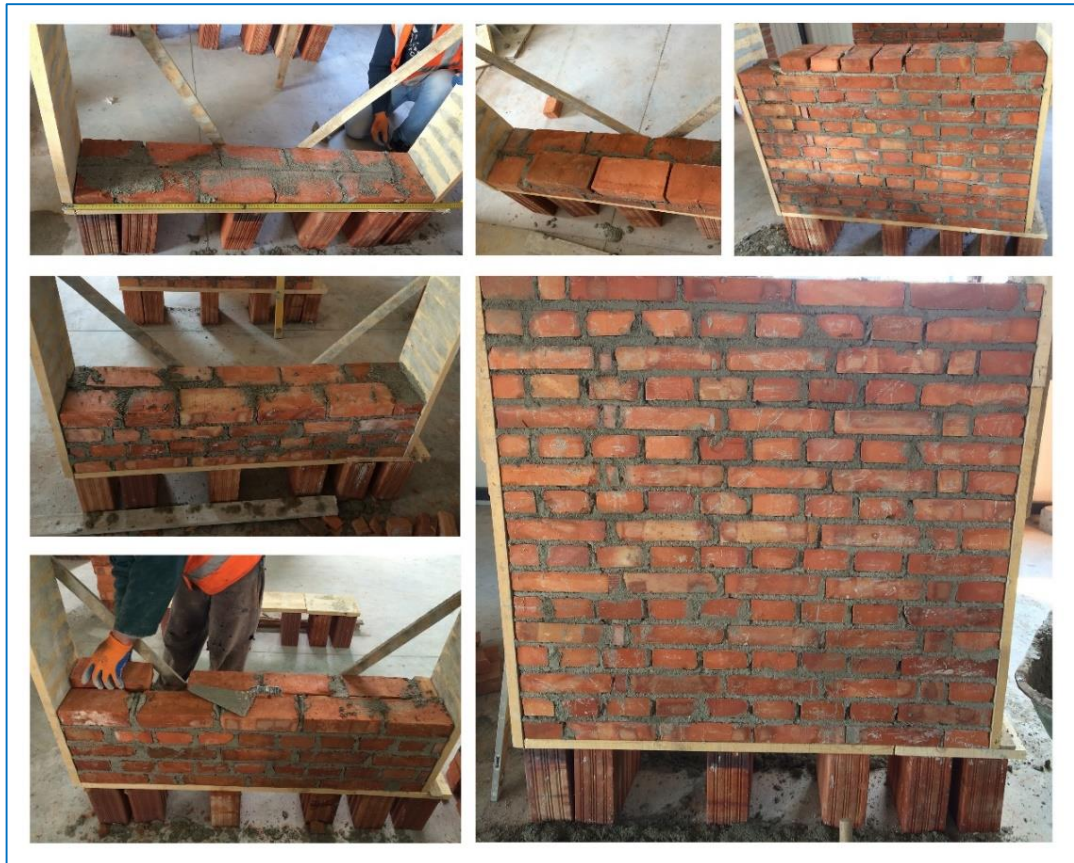
Figure 17. Construction process of plain walls.
