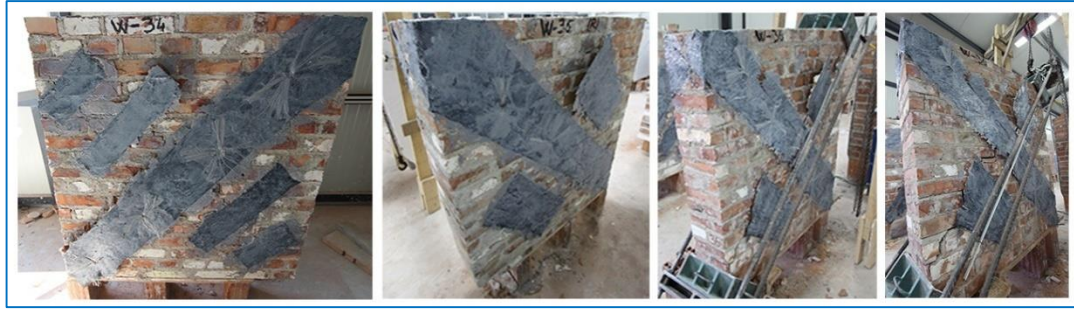
Figure 41. Failure mode of C-FRP repaired wall panels of Series 2.
