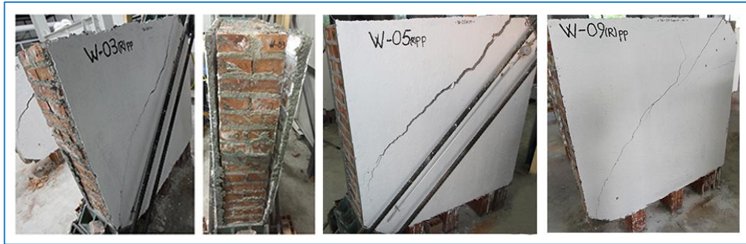
Figure 39. Failure mode of polypropylene reinforced mortar repaired wall panels of Series 1.
