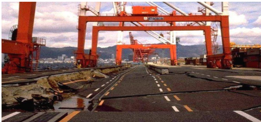
Figure 4. A considerable amount of damages on the seaport in Kobe during the earthquake in 1995 [4]
