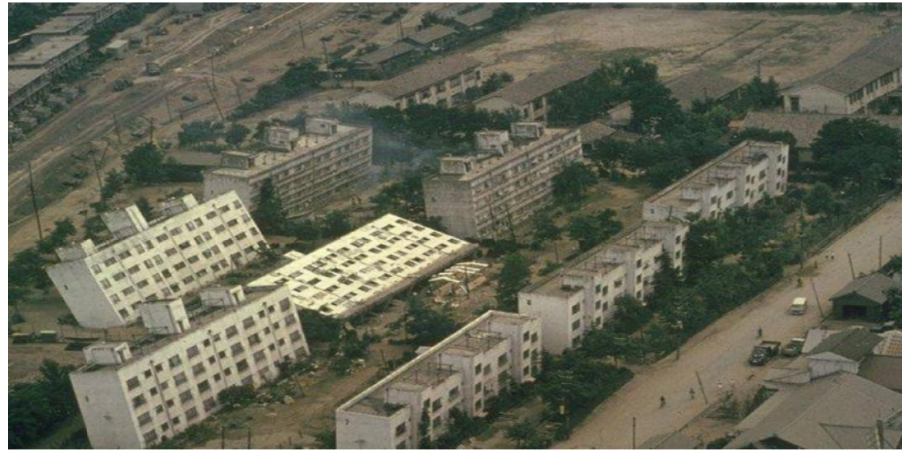
Figure 1. The apartment block destruction as the result of lateral spread, Niigata, 1964 [1]
