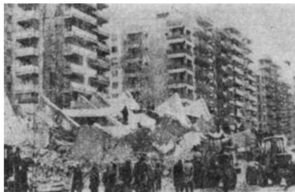
Figure 2.3 Building collapse in 1977 Vrancea earthquake WHE Report 78, Romania [11]
