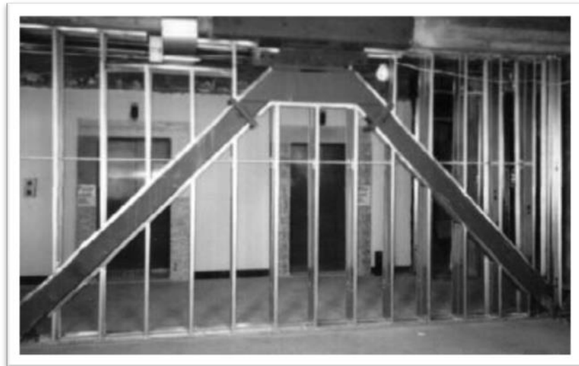
Figure 8 Friction dampers as X – brace and chevron brace, (Moe Cheung et al, 2000)
