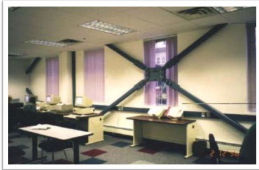
X- Braced friction damper
