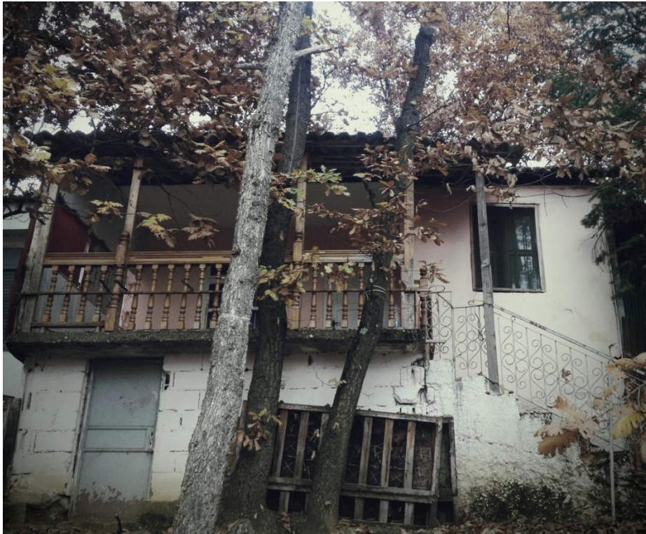
Figure 28. Nashec: House in average condition
