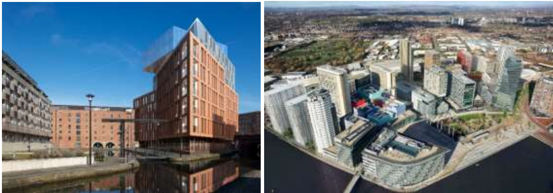
Figure 37. Building designed by Ian Simpron Architects [ Photo by Creative Heritage Consultants Ltd, Online: http://creative-heritage.net/ ]
