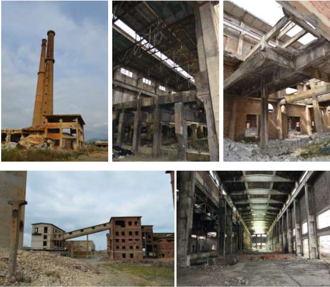
Figure 137. Laç Superphosphate Complex, September 2016 [photos by the author]
