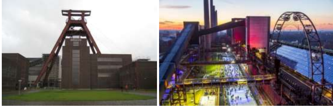
Figure 7. The Eiffel Tower of the Ruhr, part of The Zollverein Coal Mine in Essen, Germany [Chandler J., 2008] 6
