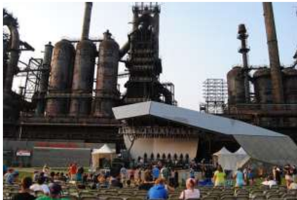
Figure 45. Bethlehem Steel Mill [ Online:
