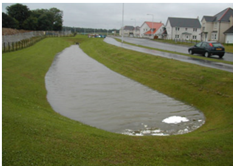
c) Temporary detention ponds
