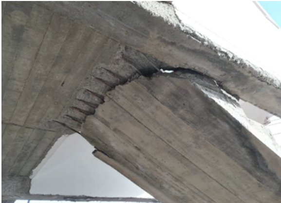
Photo 7. Wrong ladder support
