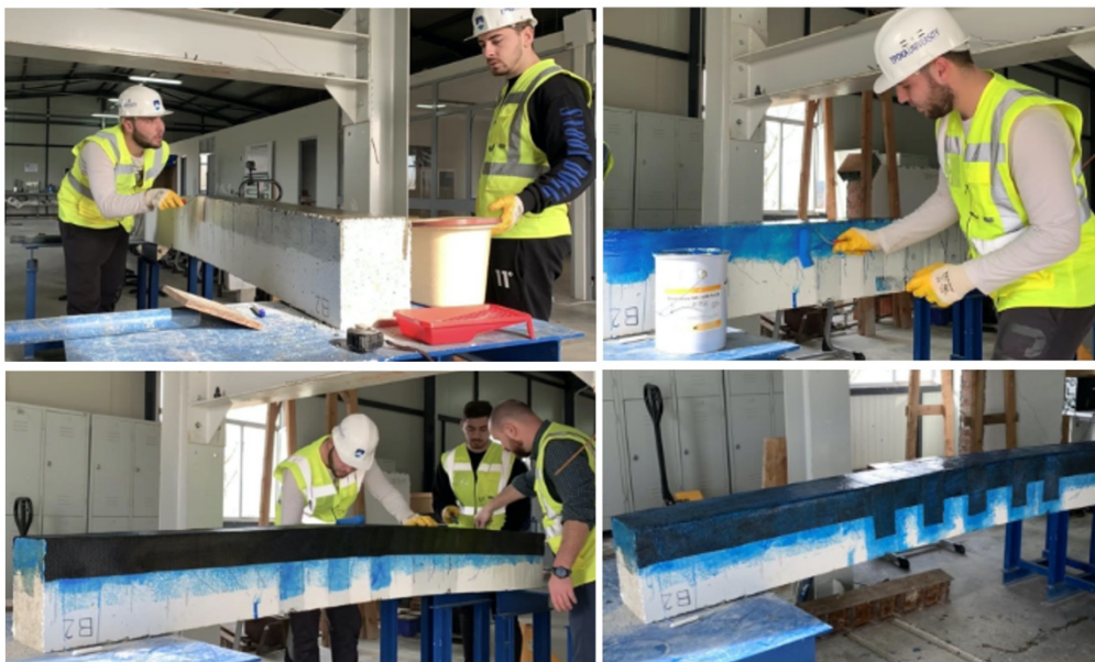
Figure 6. Application of CFRP on beam B2.
