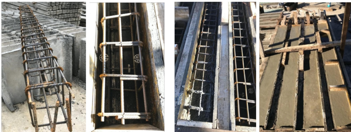
Figure 3. Step-by-step construction of the beams.
