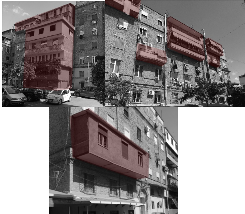
Figure 6. Informal additions in the inner facade. (courtesy of the authors)
