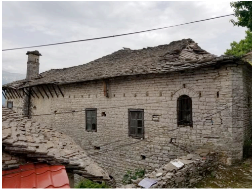
Figure 3. Roof degradation
