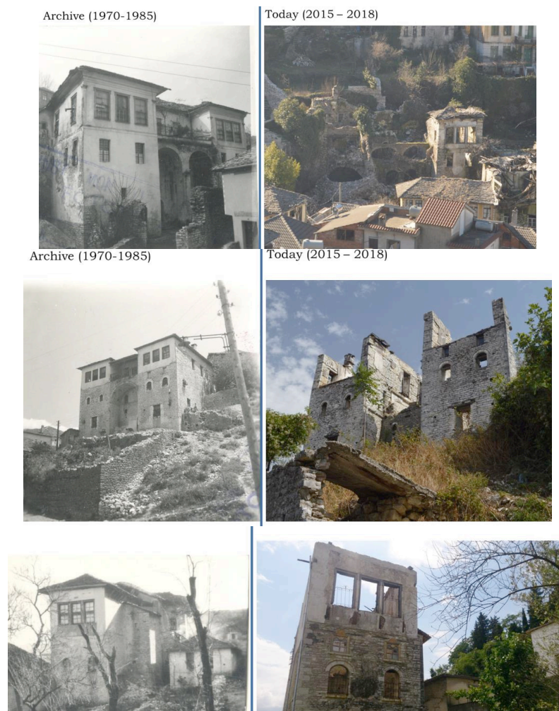
Figure 2. Degradation of dwellings in Gjirokastra [8]
