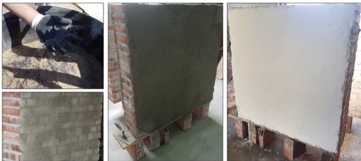
Figure 1. Polypropylene reinforced mortar coating of the URM panels.
