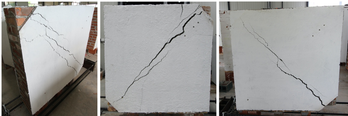
Figure 5. Failure mode of the reinforced panels.
