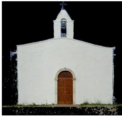
Figure 1: photopiano processing of the church of San Michele in Frangesto, Fasano
