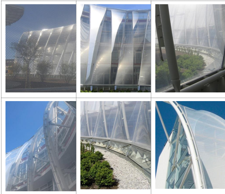
Figure 8: Figures of Gerontology technology center in Bad Tölz from inside and outside the double skin facade. ( www.kochmembranen.com 2017)
