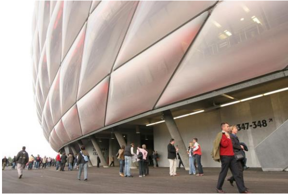
Figure 2: Allianz Arena Stadium in Munich ( www.to-experts.com 2017)
