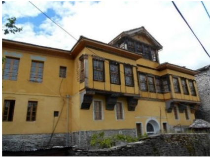
Figure 32: Fico facade painted in mustard colour in the outside: the upper windows are bigger
