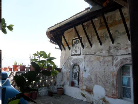
Figure 30: Roof construction element in Zekate House
