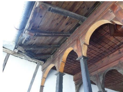
Figure 25: Roof construction element in Zekate House
