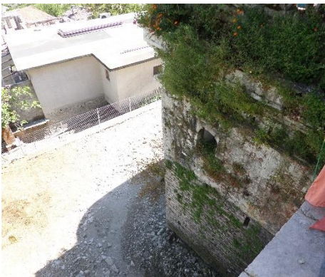
Figure 27: The greenery used in the walls of the Kikino house
