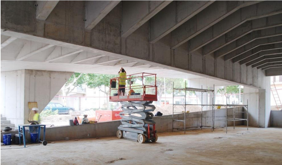
Figure 5: Concrete beams of the new hall supporting the new square (the roof of the hall).
