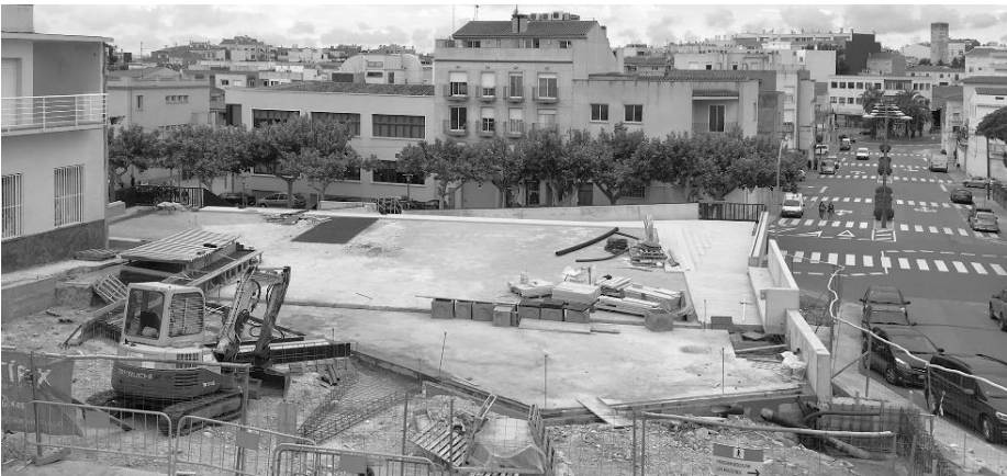
Figure 6: The roof of the new Hall (the new square).
