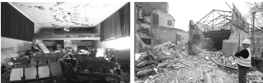
Figure 3: 2014, demolition of the old Parochial Hall.
