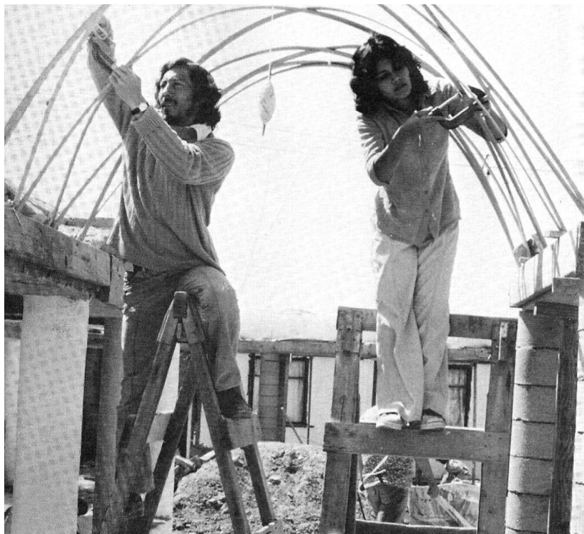
Fig. 8: Dwellers building their house (source: Alexander, 1985: p. 296).
