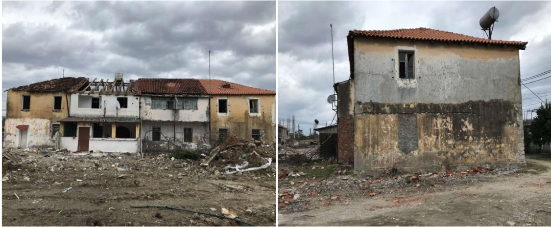
Figure 259: Building nr.7 in street "Rira" in Thumane of template A2
