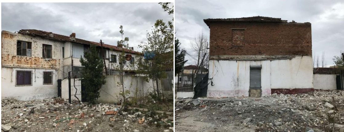
Figure 261: Building nr.13 in street "Rira" in Thumane of template A1
