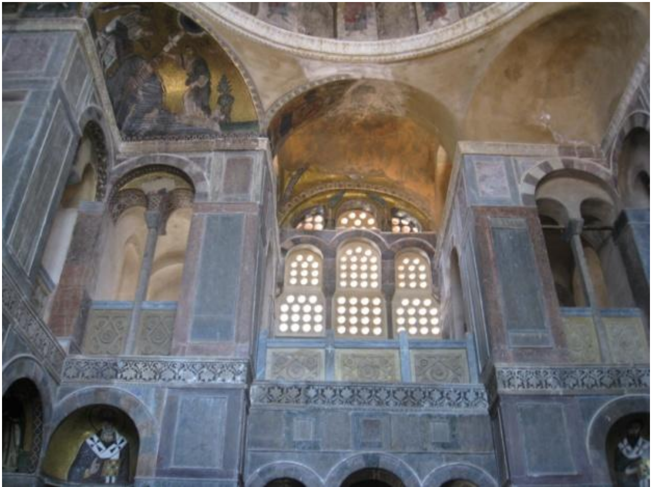
Fig. 4: The mosaics and marble claddings as representational elements which convey a symbolic meaning and which reveal in a discreet manner the constructive logic of the structure. Catholicon of Hosios Loukas monastery, Greece, 10 th -11 th century.
