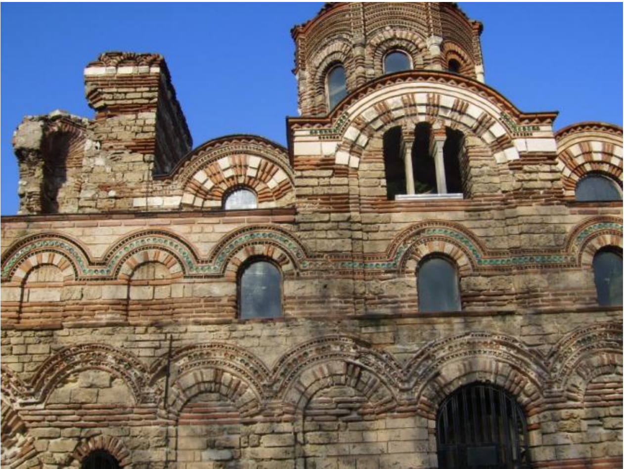
Fig. 8: Atectonic or the manneristic subversion of structural clarity in Byzantine architecture: Pantokrator church in Nesebar, Bulgaria, 14 th century. Detail of south façade showing the tiers of decorative arches with out-of-step rhythms. Some of the arches have a correspondence with structural arches inside, but most do not.
