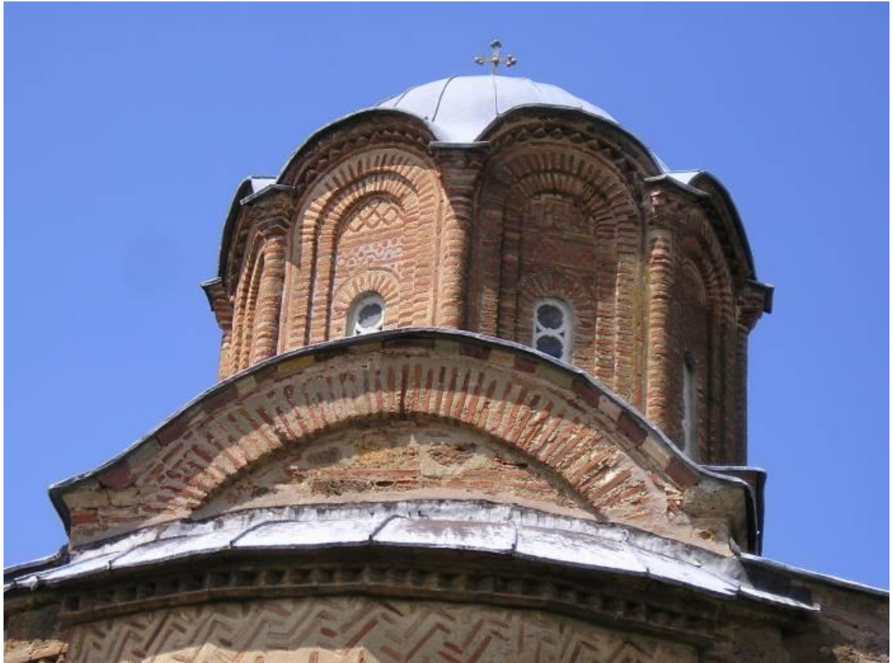
Fig. 2: The exterior surface of the wall and the roofing as cladding-like elements which reveal the constructive logic of the structure. Church of Lesnovo Monastery, Macedonia (former Yugoslavian republic), 14 th century.
