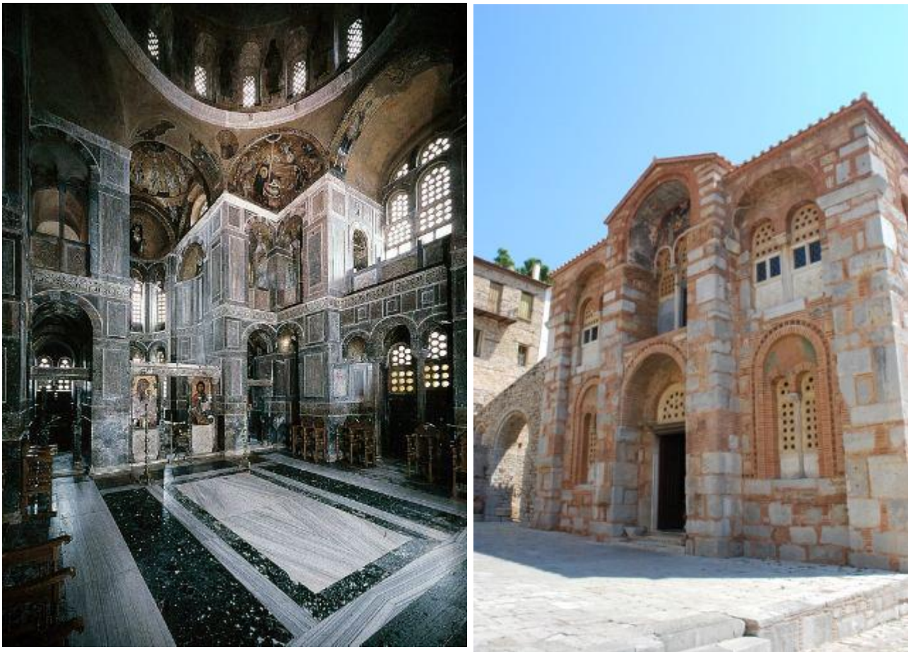
Fig. 5-6: Tectonic or structural clarity in Byzantine church architecture: Catholicicon of Hosios Loukas monastery, Greece, 10 th -11 th century.
