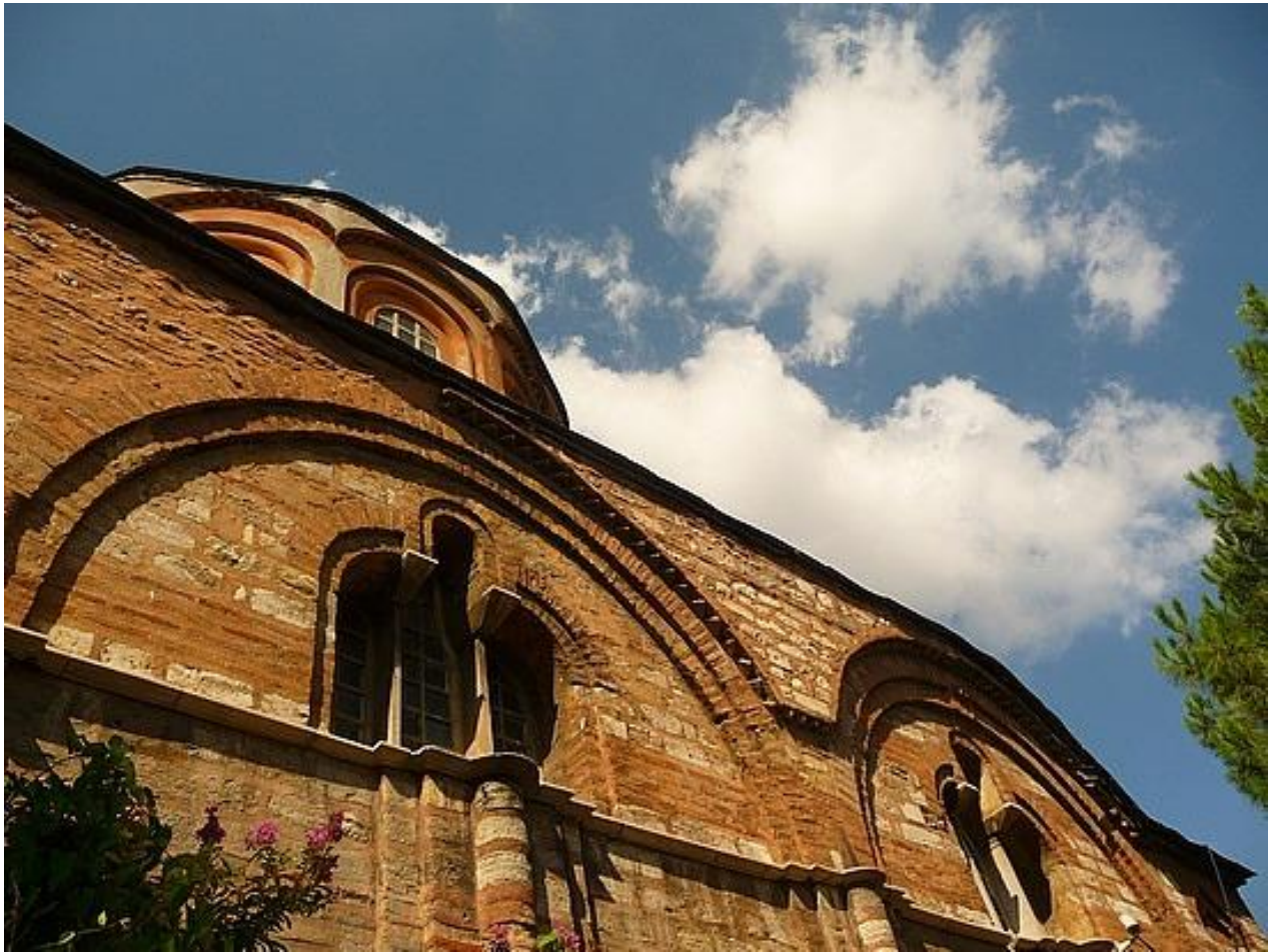
Fig. 7: Atectonic or the manneristic subversion of structural clarity in Byzantine architecture: Monastery Savior in Chora, Constantinople, south façade (of the parekklesion ), 14 th century. Detail showing how identical elements seem to carry the springing of decorative arches and the windows at the center of the arches.
