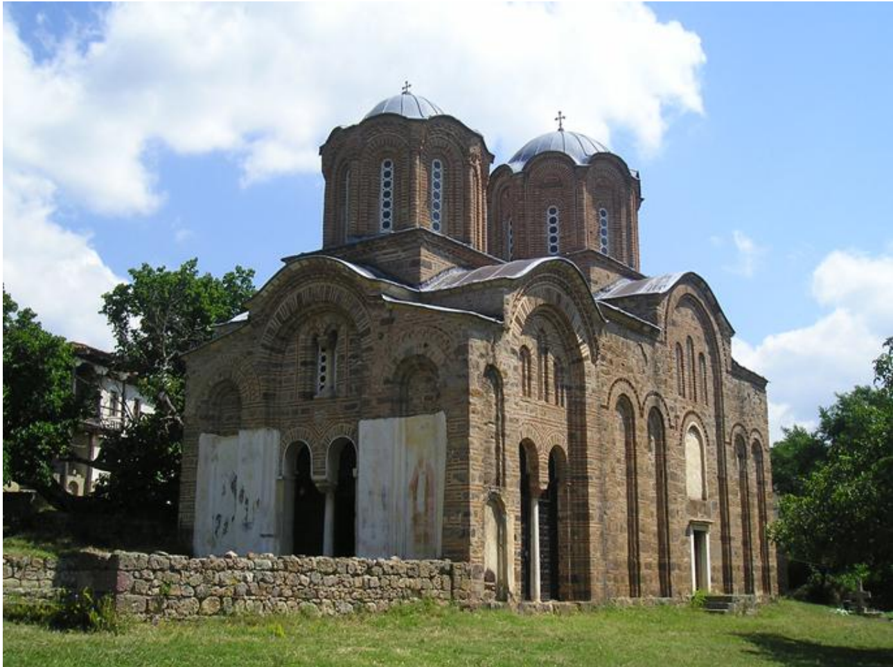
Fig. 1: The decorative masonry and roofing as the art form which represents the core form (load-bearing structure). Church of Lesnovo Monastery, Macedonia (former Yugoslavian republic), 14 th century.
