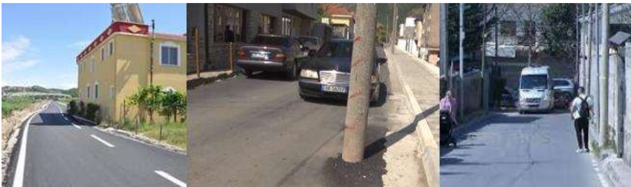
Figure 3. Some road/street views in Albania
