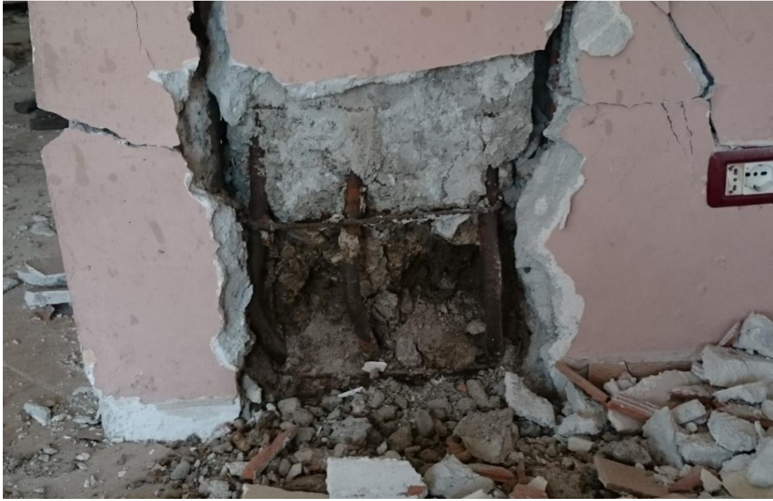
Figure 26: Column failure, corroded rebars, poor concrete
