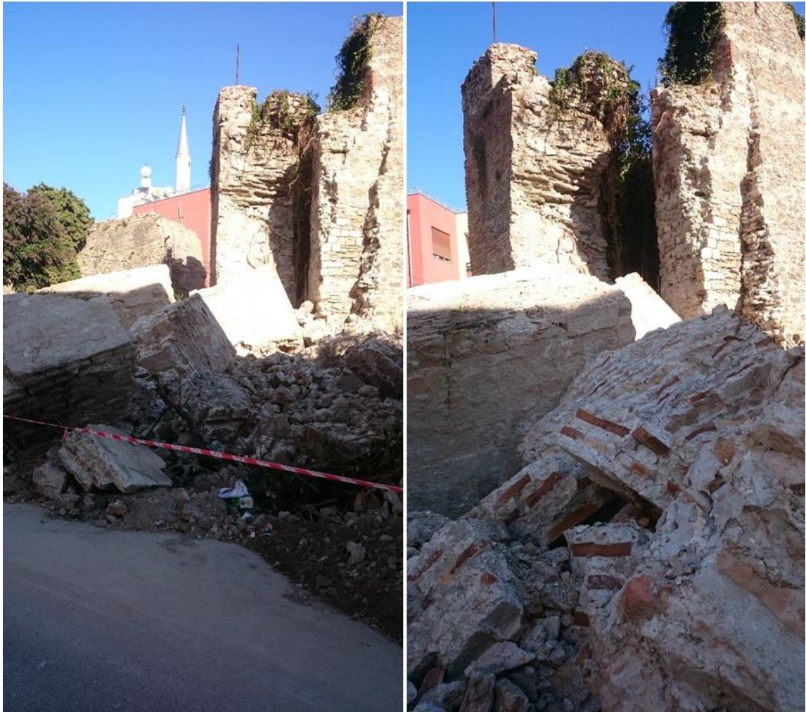
Figure 53: Massive destruction of the outer walls of the ancient castle
