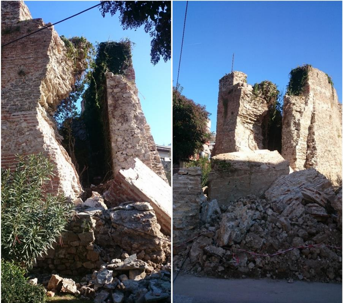
Figure 52: Heavy damages in the fortified walls of Durrës Castle
