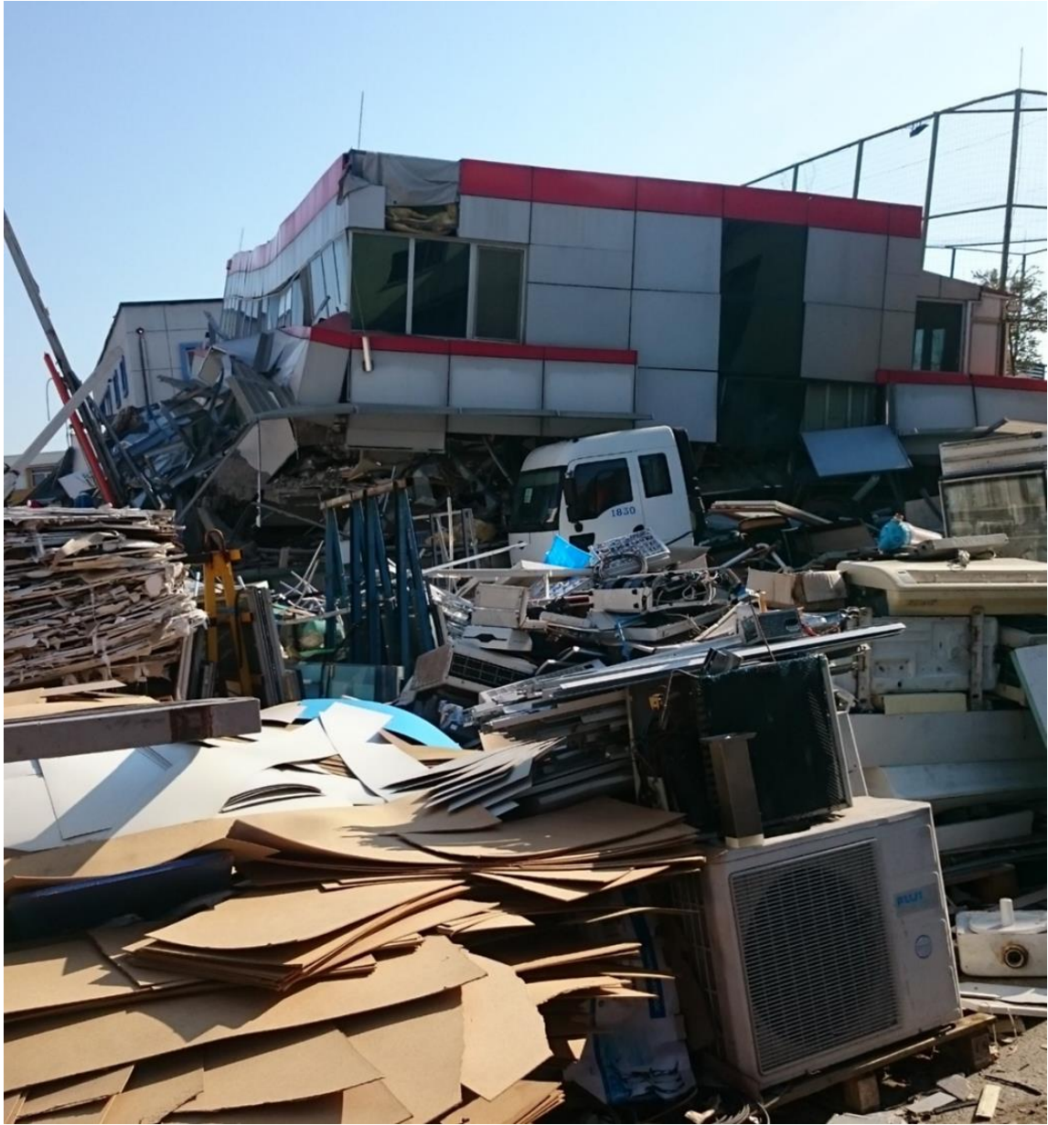
Figure 13: Building collapsed completely
