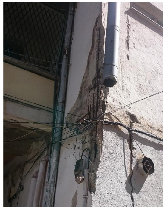
Figure 26: Column failure, corroded rebars, poor concrete
