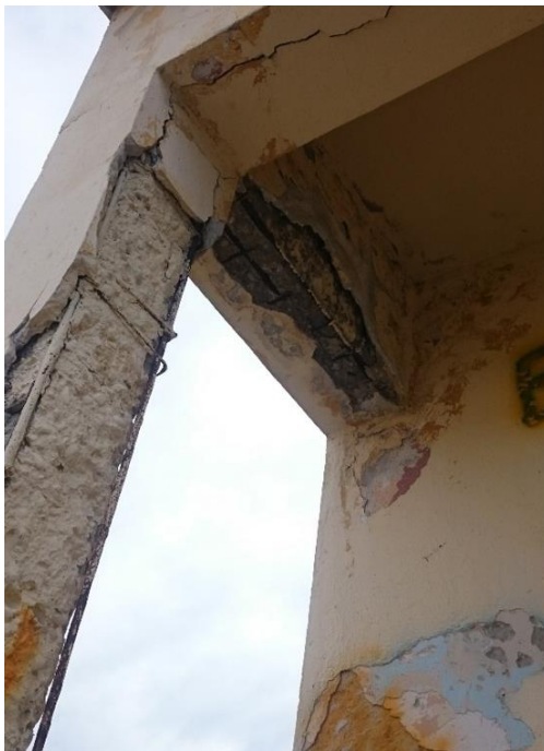
Figure 27: Damaged corner column, corroded bars
