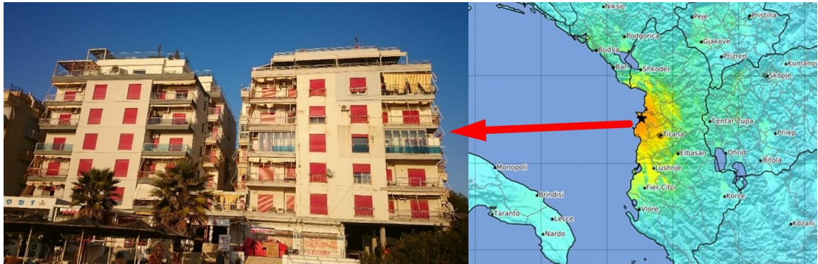
Figure 78: Location of E Template buildings at Iliria beach in Durrës, close to November 26, 2019 epicenter
