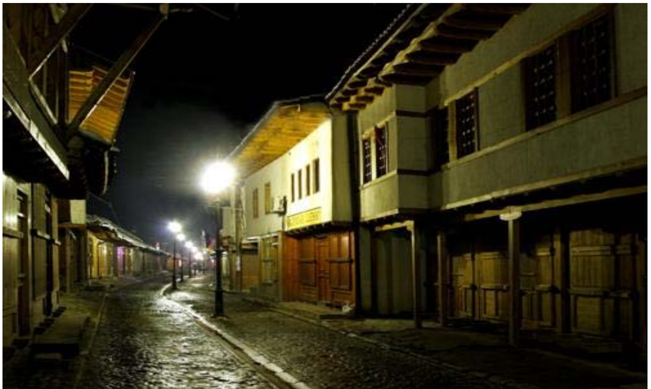
Fig. 10 Reconstruction of the Old Bazar in Gjakova, 2003 (greengopost, 2011)
