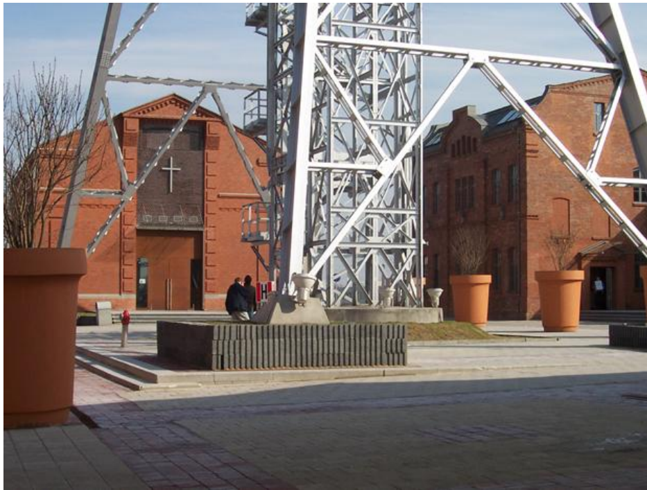
Fig. 2: St. Barbara Chapel in the Silesia City Center, an adaptation of the hoist machine building. In the foreground is the basis for the construction of the tower shaft Georg. Fig. Thomas Wagner.
